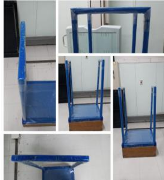
Figure 10 - Final repair of the supports
