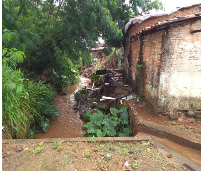
Figure 1: Disposal of domestic sewage into Tanque stream
